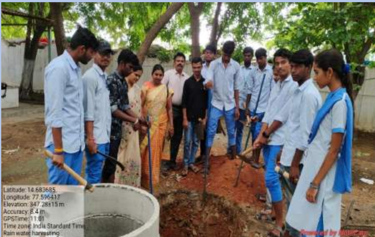
Construction of Recharge pit near the borewell
