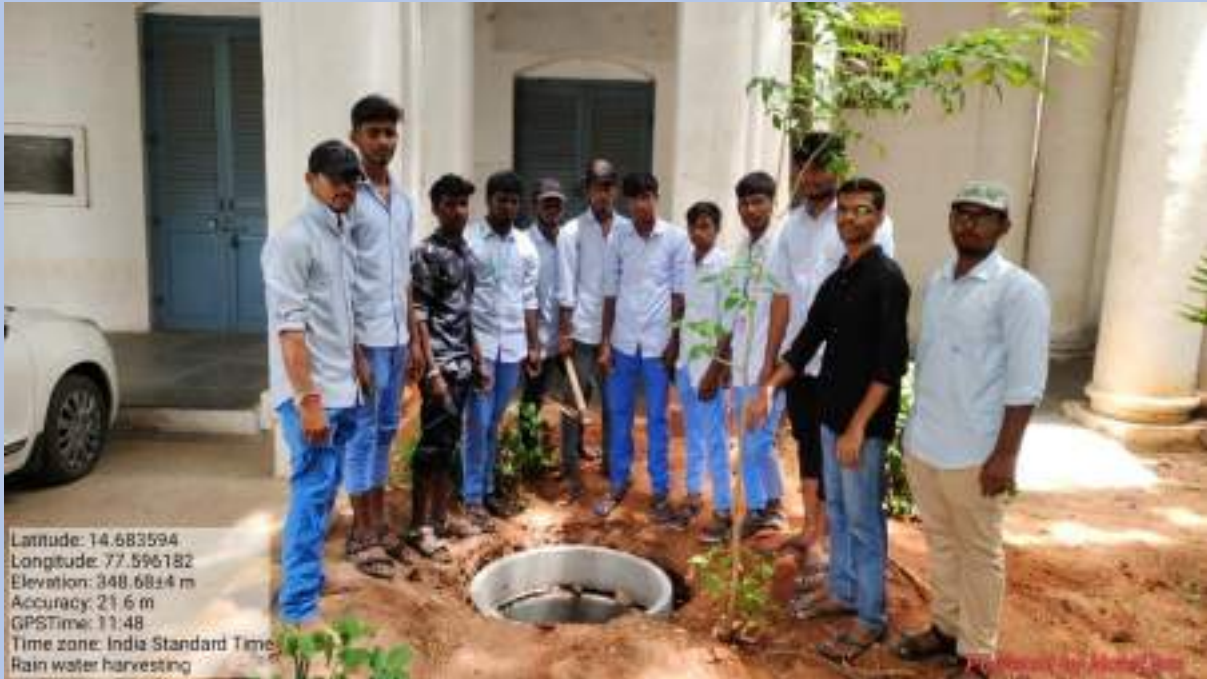
Construction of Percolation pit to harvest rain water
